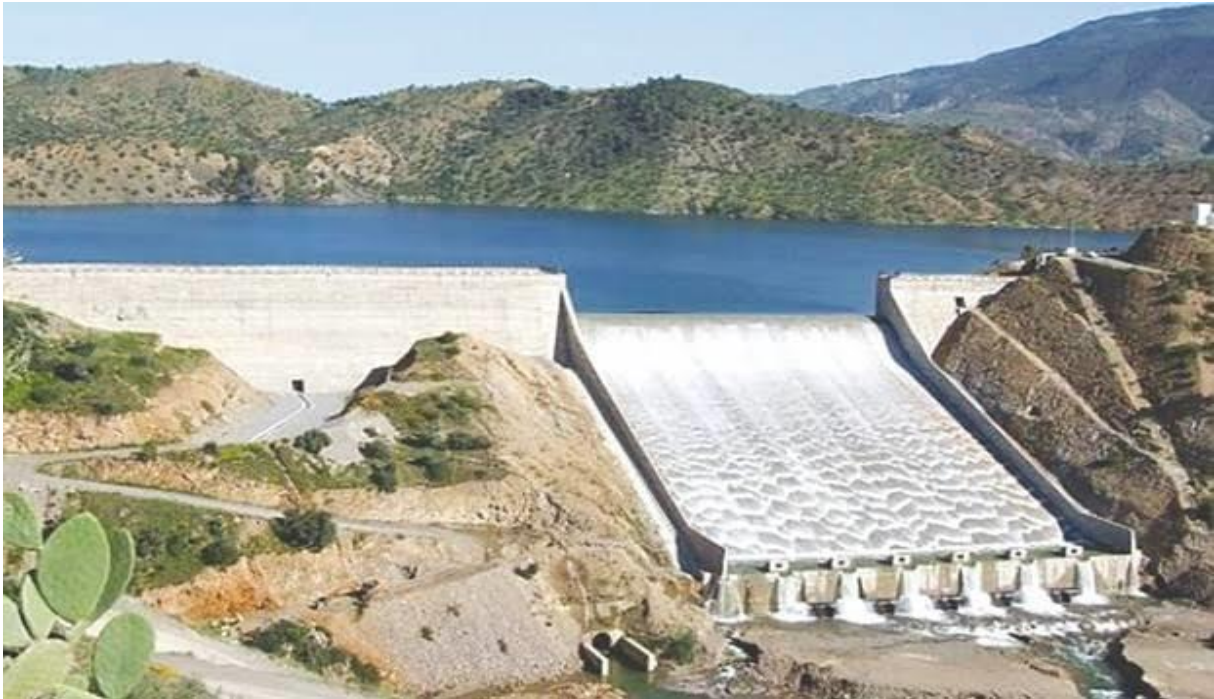
Figure (I-6): Barrage de Tichy-Haf
