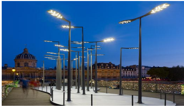
Figure 41: L'éclairage public Source : https://www.eclatec.com
