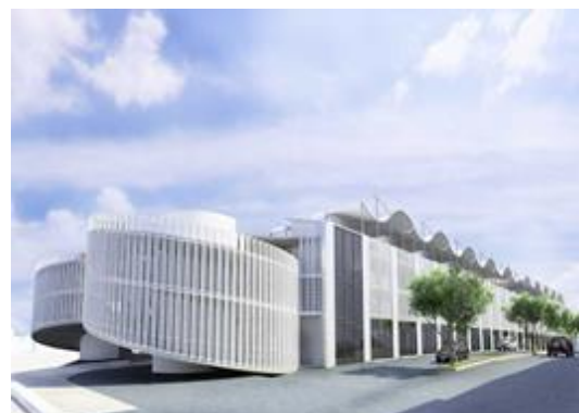
Figure 12: parking a étage.
