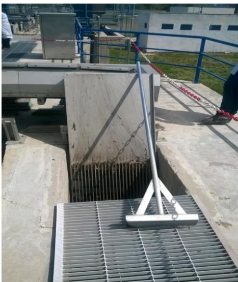
Figure I-3. Grille manuelle STEP SET.
