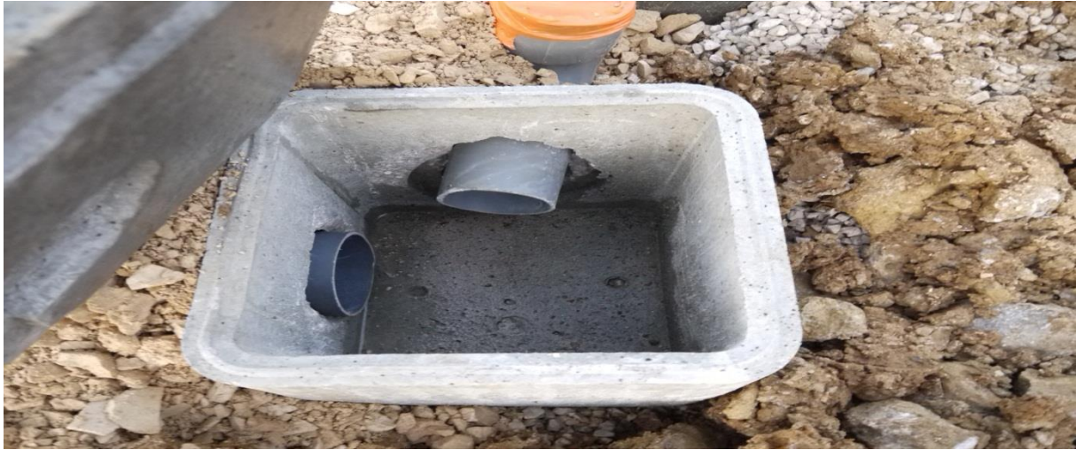
Figure V.6: Regard de branchement
