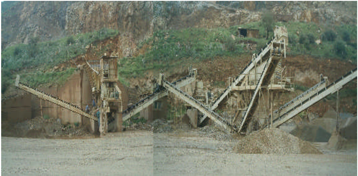
Figure (III-3) : Station de concassage de la SOMACOB AKBOU.
