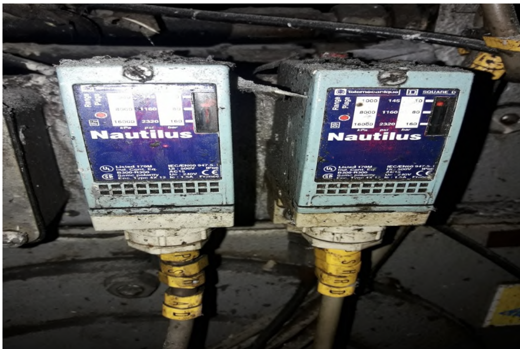
Figure I. 9 Pressostat
