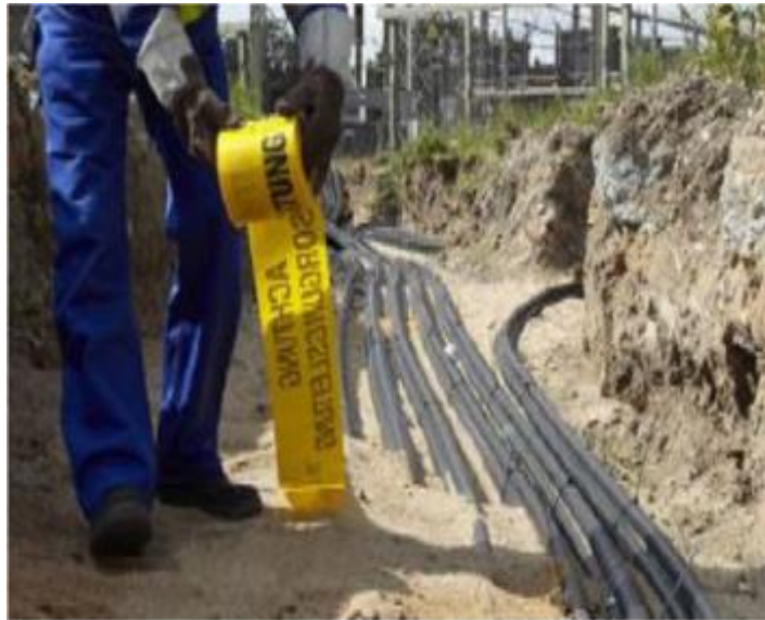
Figure I.12: des câbles souterrains.
