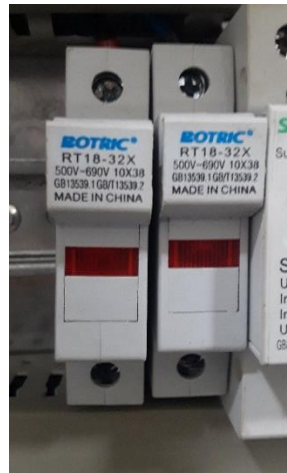
Figure III.18: Porte fusible
