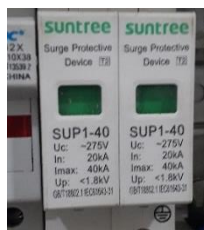
Figure III.19 : Parafoudre AC
