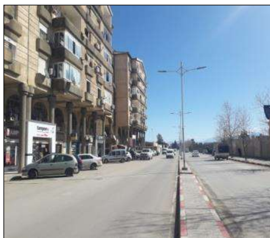
Figure 97 : Route Bounadaoui Nacer
