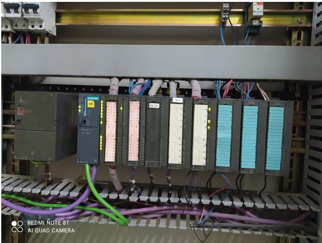
Figure II.15 : Architecture réelle Automate SIMATIC S7-300
