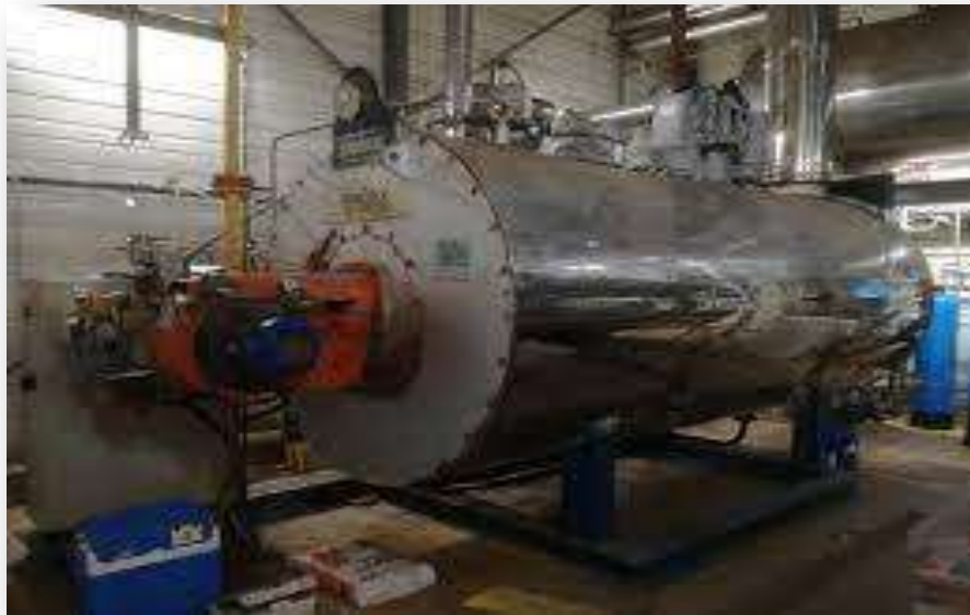
Figure. II.11. Chaudière
