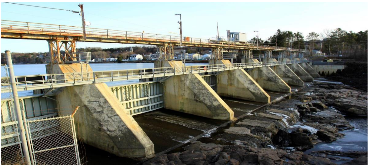
Figure II-8 Barrage mobile du Melville, Canada [13]
