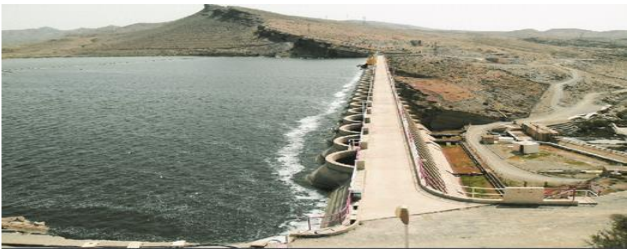
Figure II-6 Barrage a voutes multiples , el ksob ,Algérie [11]
