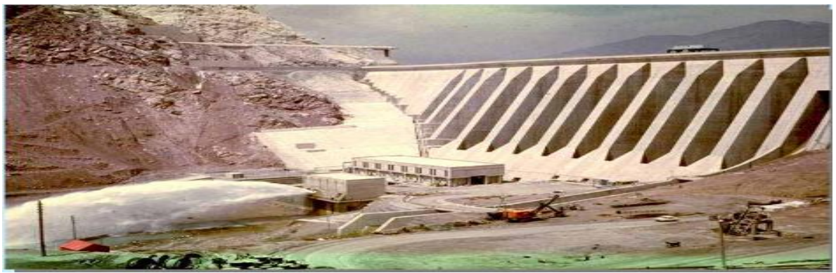
Figure II-4 Barrage latiyen, Iran [9]
