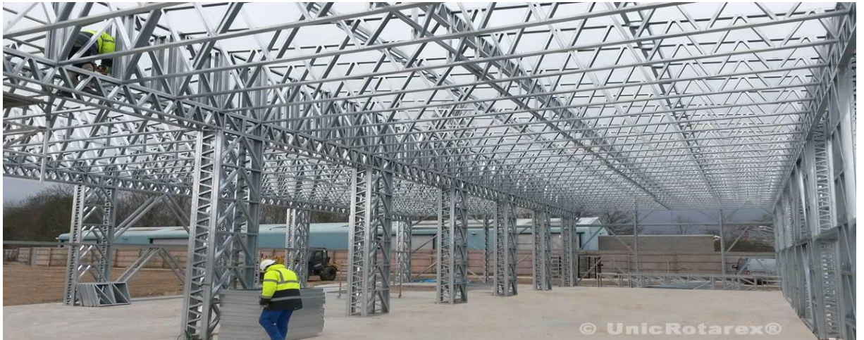
Figure I.4: structure en treillis
