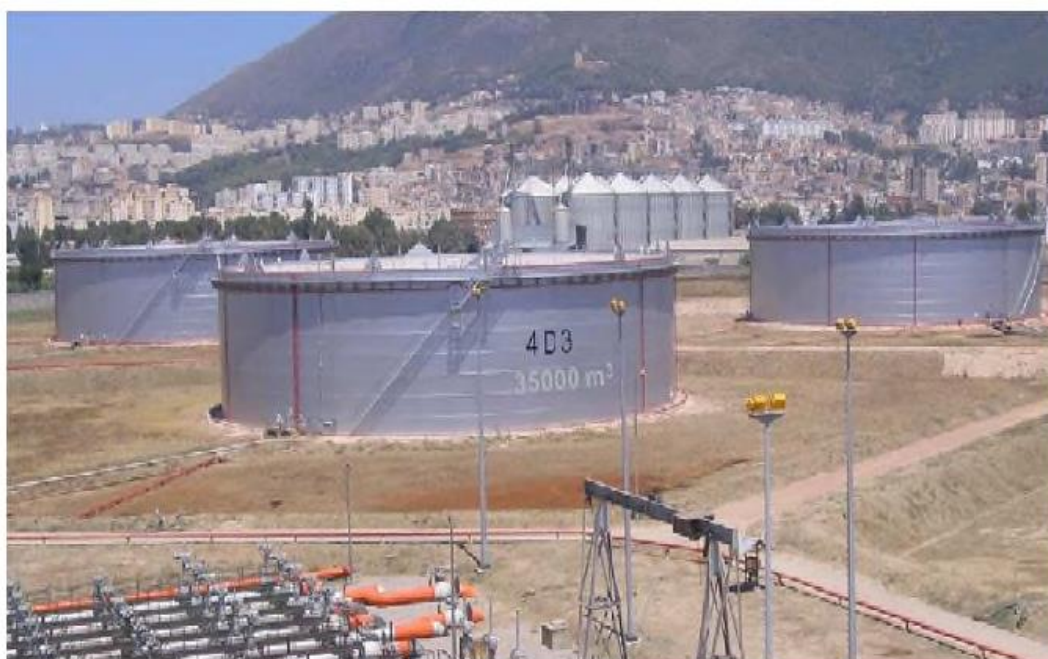
Figure II-3: Parc de stockage
