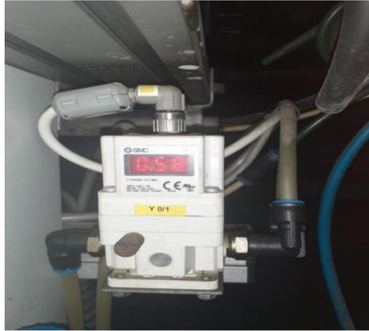
**Figure 1.14 :** Electro pneumatic regulator Marque SMC Série ITV1000
