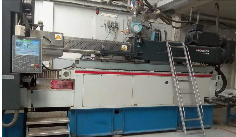
Figure III.34: Le corps du four.
