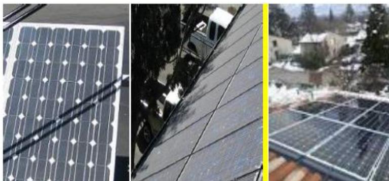
Figure I-23. L'ombrage photovoltaïque
