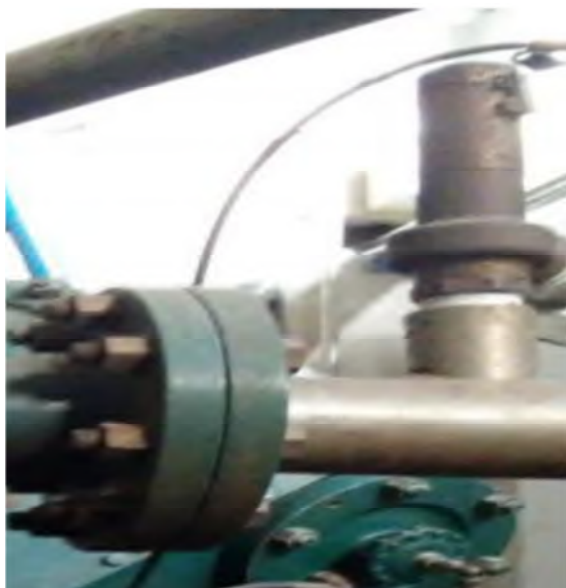
Figure II.I.17: soupape de sécurité
