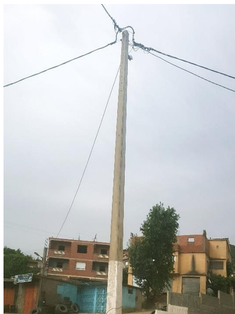
Figure 17: Support en béton armé
