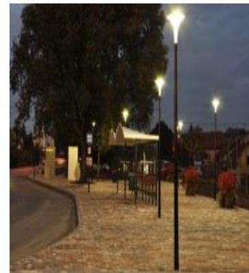
Figure 1. 9: luminaire Source : www.google.com
