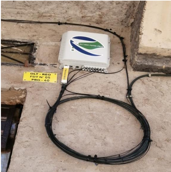
Figure II.23: PBO extérieur.
