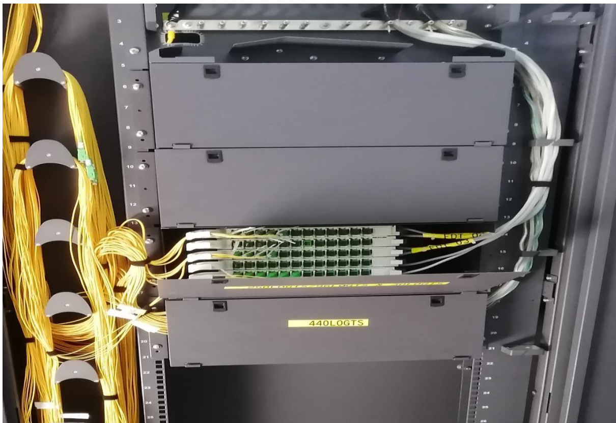
Figure II.12: Façade passive (ODF 288).
