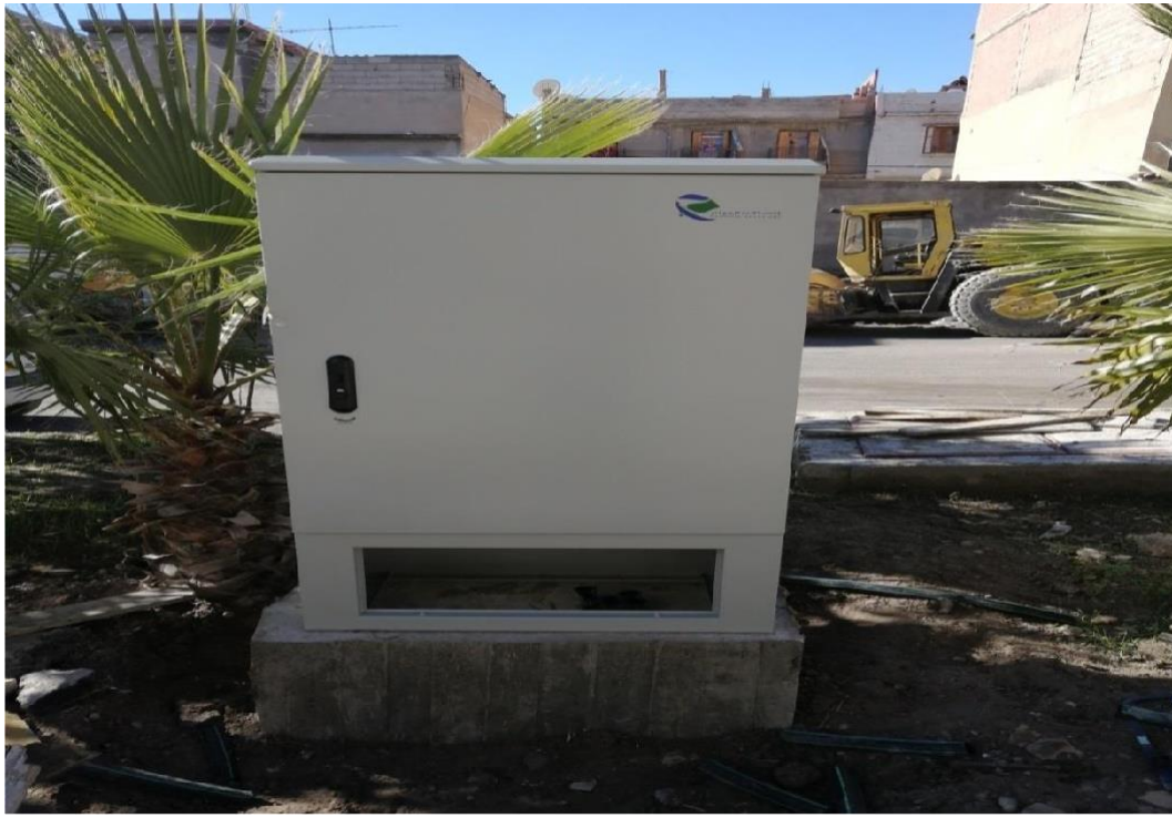
Figure II.16: FDT (Fiber distribution terminal).
