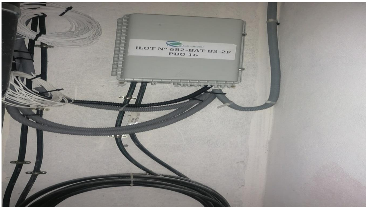
Figure II.21: PBO intérieur.
