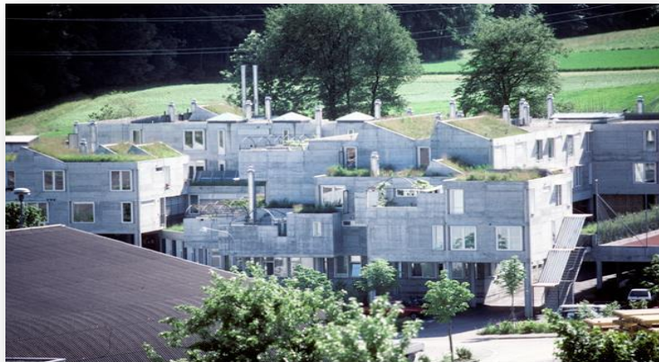
Figure 20 : villa urbaine, source: (Bougui & Abour, 2017-2018)
