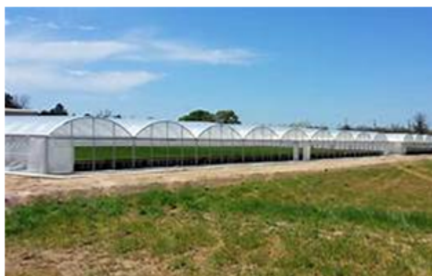
Figure 1.5 : Serre tunnel spid.
