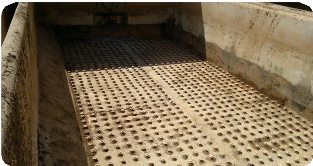
Figure (III.16) : Le lit filtrant
