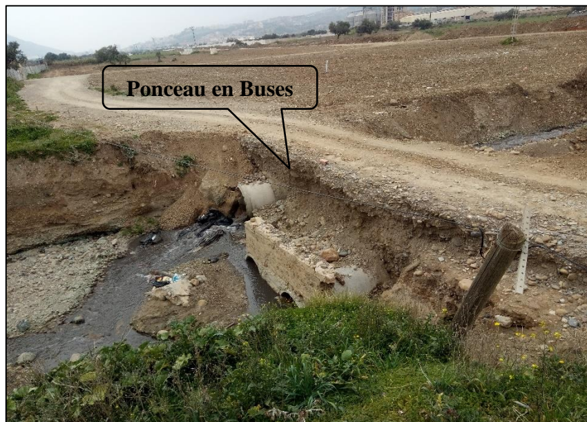
Figure (III.14) : Ponceau traversant oued TIFRIT. (Ph. Prises le 28/05/2022).
