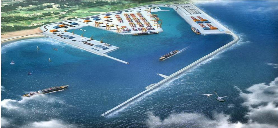
Figure 7: Le port de Djendjen
