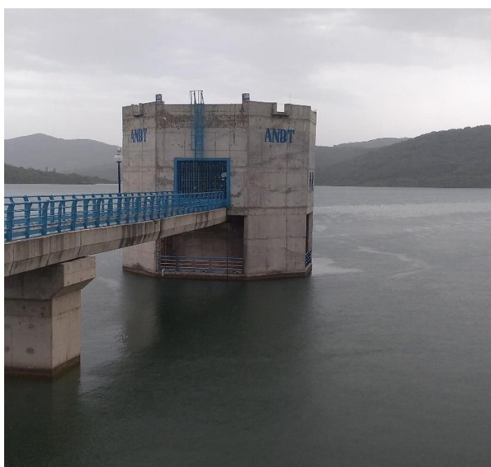
Figure 16: La tour de prise
