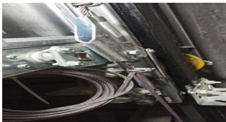
Figure I.11 : Parachute
