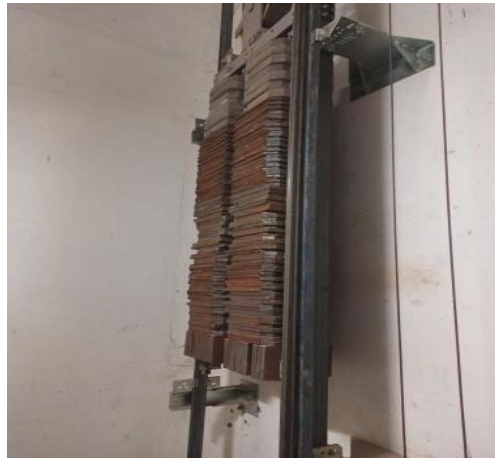
Figure I.12 : Le contrepoids
