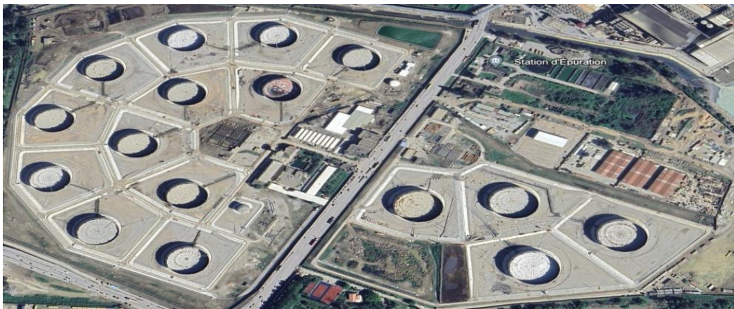
Figure I.2 : Terminal marin de Bejaia.
