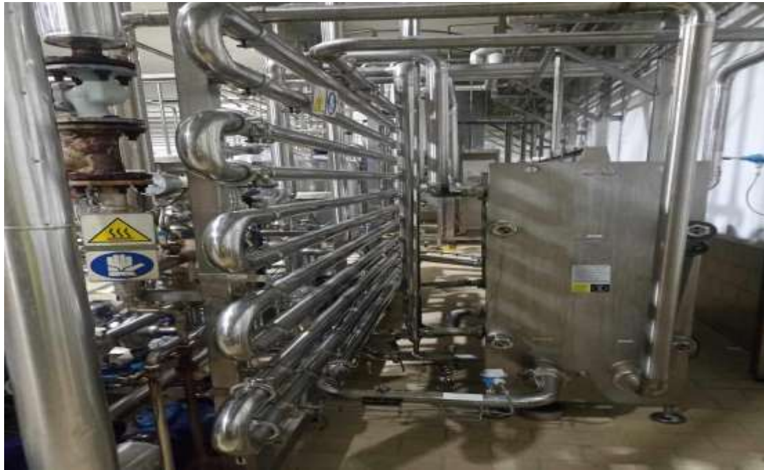
Figure II.5: Echangeur coaxiaux (double tube) CEVITAL
