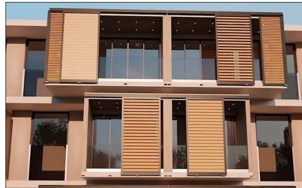
Figure 28: brise soleil en bois verticale orientable (Source : https://www.glass-systems.fr , 2024)
