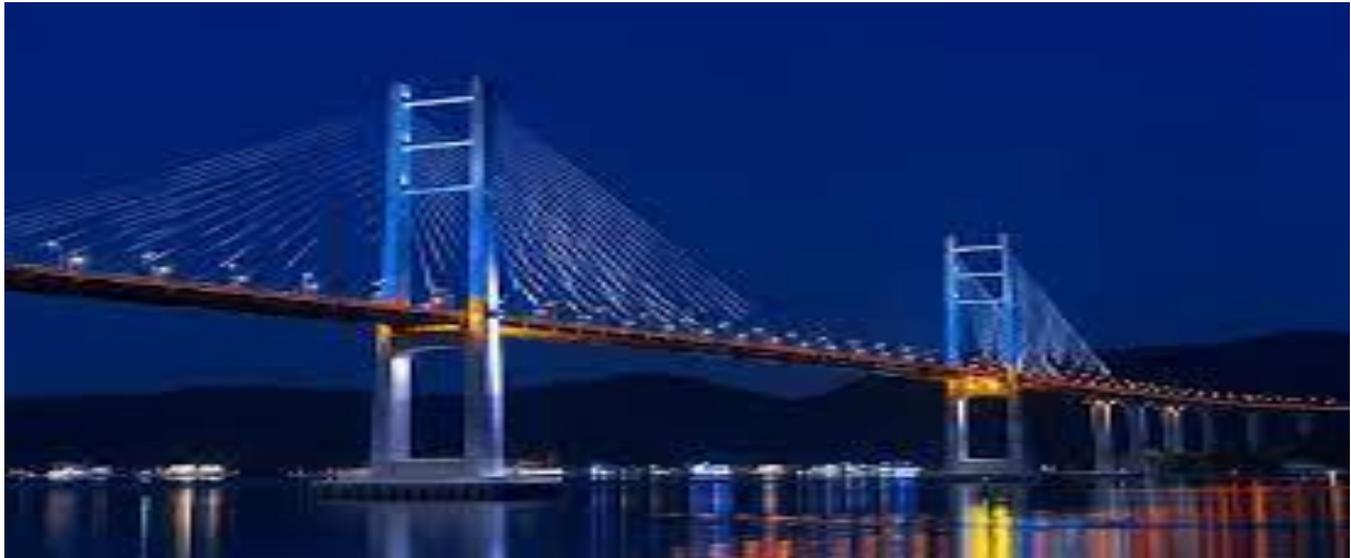
Figure I.5 pont a haubans[1]
