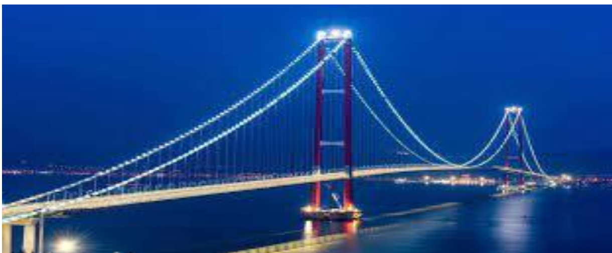
Figure I.3 exemple pont suspendu[1]
