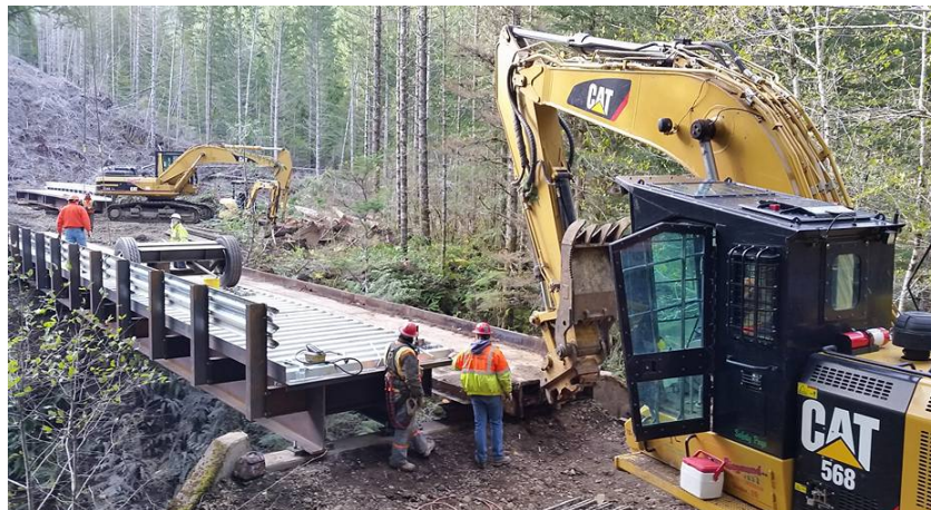
Figure 1.4 – Road construction and upgrading operation (source:[25])
