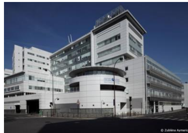
Figure I.8: Hôpital George Pompidou Source: www.castelalu.fayat.com
