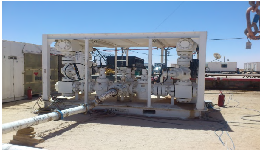
Figure III.11 : Semi Auto Choke. [8]
