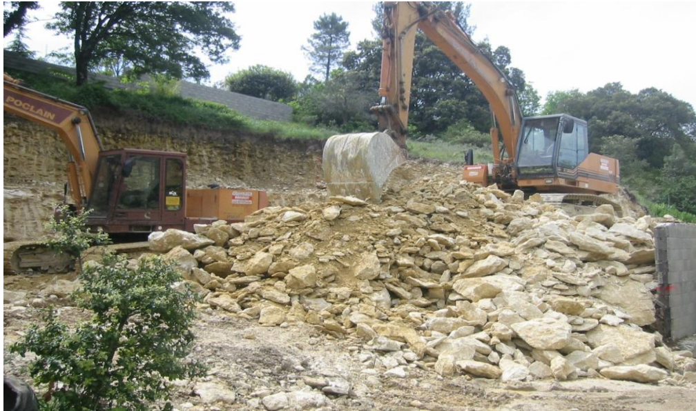
Figure II.2: Travaux de terrassement [4]
