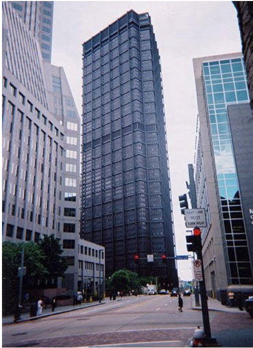
Figure I.32: US steel building , Pittsburgh, USA, 1967
