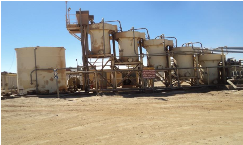
Figure II.7: Colonnes de charbon. [Photo prise]
