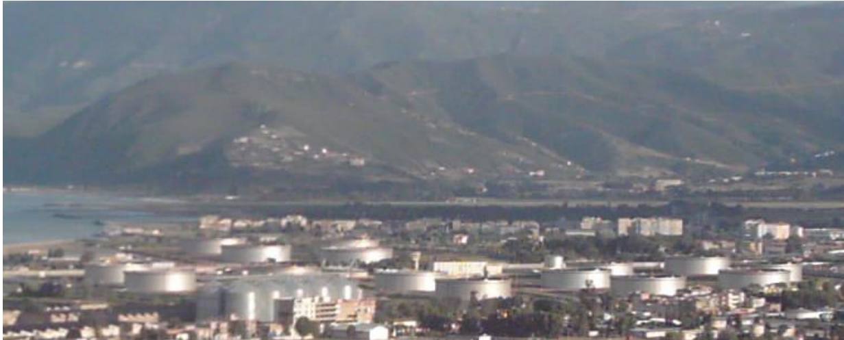
Figure I.11. Terminal Marin de Bejaia.
