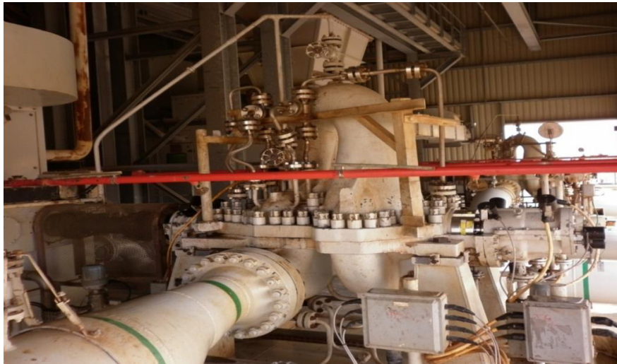
Figure II.4 : La pompe centrifuge BF 10X18 BFD.
