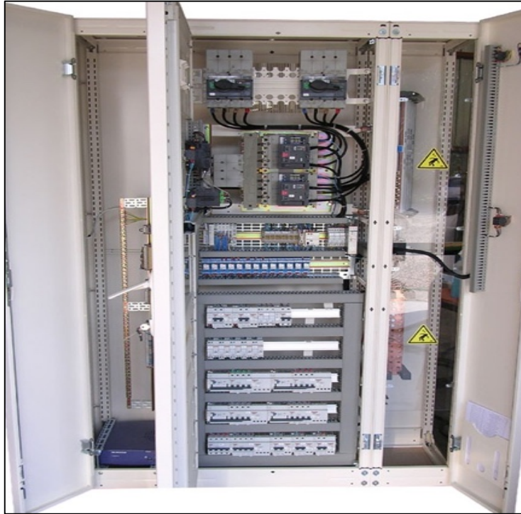
Figure II.22. Exemple d'armoire TGBT
