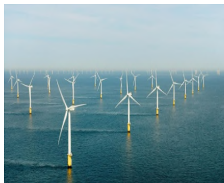
Figure I 6. Eoliennes Off shore
