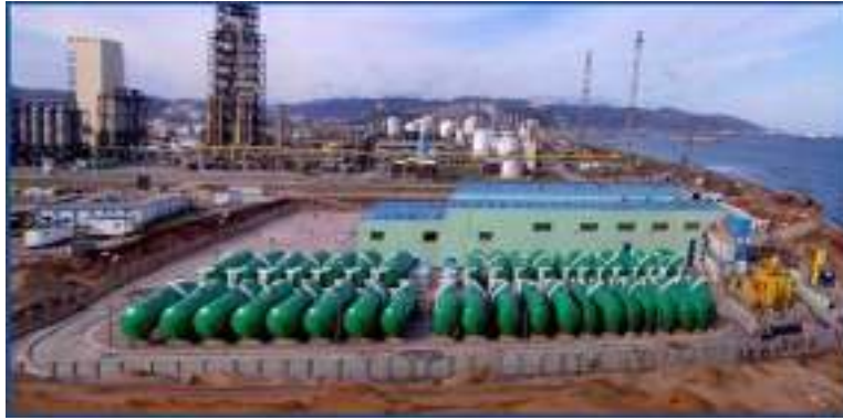
Figure III.1: station de dessalement cap Djinet
