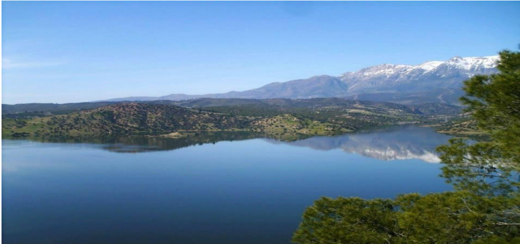
Figure 2. Photo de barrage TILES DIT.
