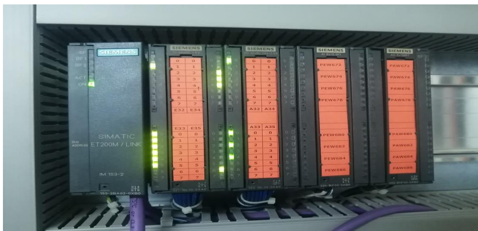
Figure III. 19 : Automate programmable ET200
