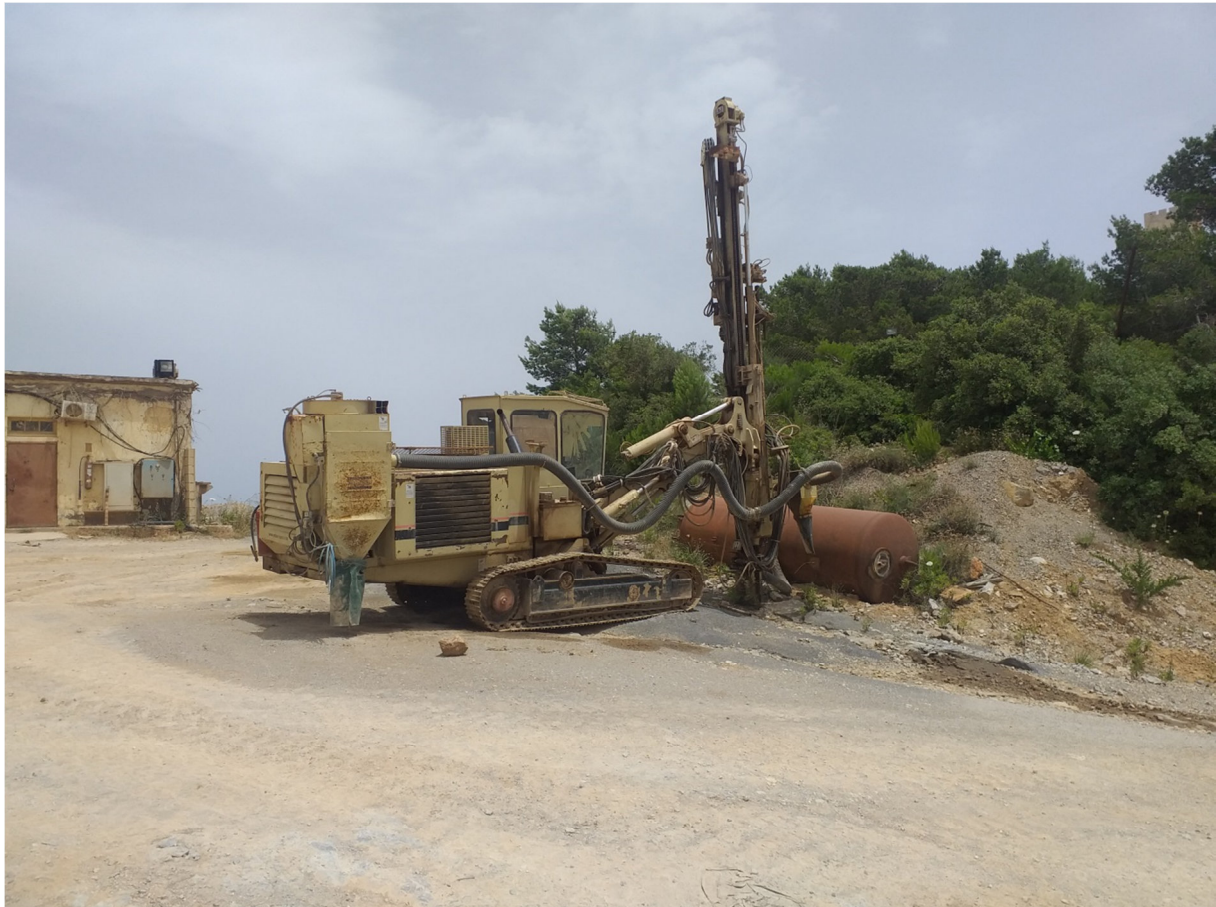
Figure III.5. Sondeuse ATLAS COPCO.
