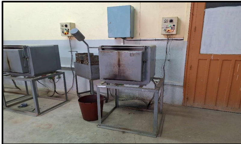
Figure II.13 : four du hall technologie
