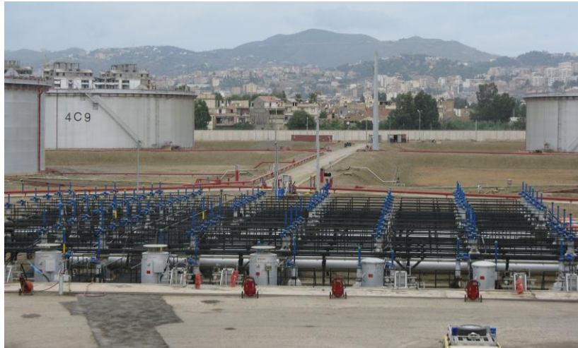
Figure I.4 : Manifold.
