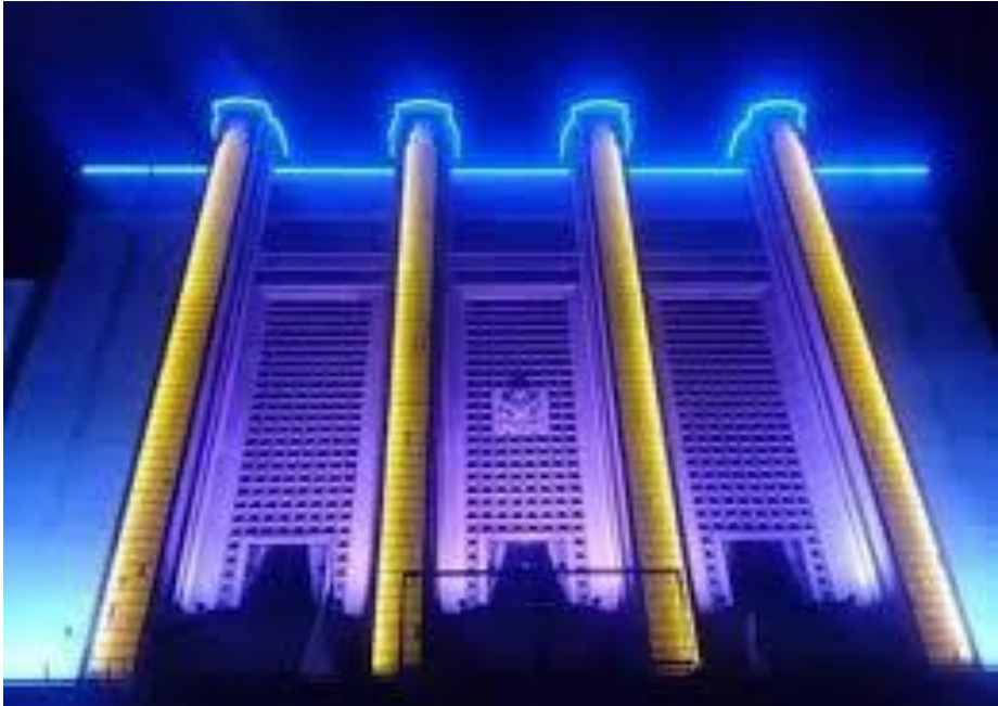
Annex 05: The front of TRB building
